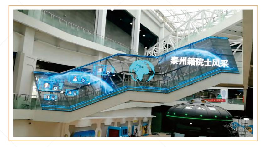
The glass-covered bridges in the Taizhou Science and Technology Museum are mostly irregular in shape and are composed of a combination of quadrilateral regions. The area and the degree of distortion are not the same. This poses a significant obstacle to the installation of display screens.
