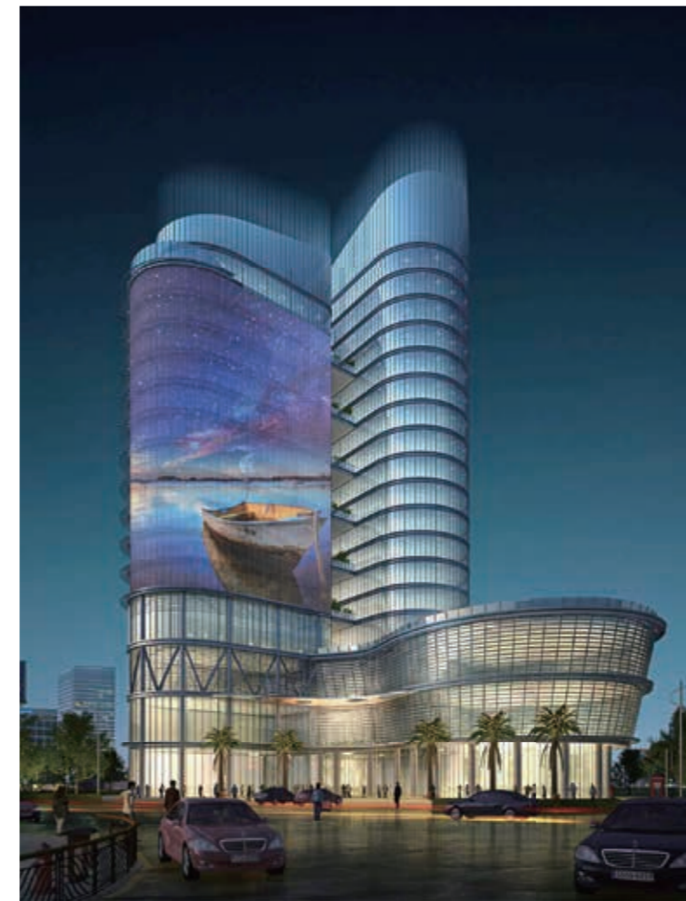
楼宇外墙 Glass facade
